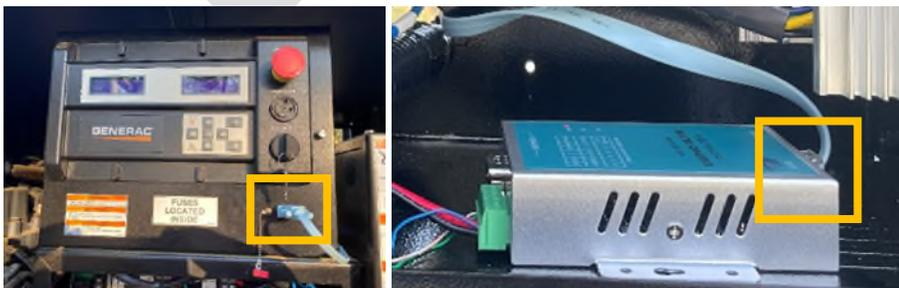
9.4. IS 9VDC-30VDC SUPPLIED TO THE MOD-RS485-CNV-10XN ON THE DC+ AND DC- CONNECTIONS? (MEASURE THE WITH A MULTIMETER)
