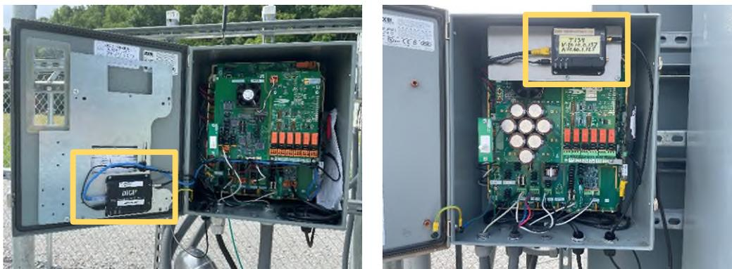
3. Remove the lighting system modem (Location shown above).
